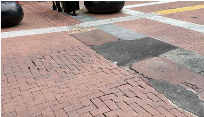
The failed drainage runnel, which was acting as an edge restraint (unintentionally), has allowed the brick paving field to begin to move as there is no firm edge available. However, note that the brick are still serviceable even though they have begun to become unstable. Tightly packed sand swept joints may have helped protect against some of this movement.
