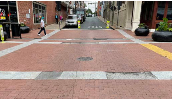
Photograph of the 4th Street East vehicular crossing indicating the serviceable and sound condition of the vast majority of the brick pavers.
