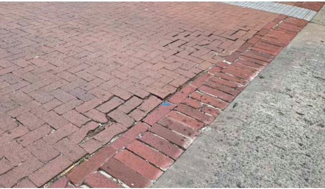
Salvaged brick banding adjacent to the concrete speed hump. Note the broken mortar, disheveled brick orientation (due to movement) and the brick paving field beginning to deflect as a result of the failed edge restraint.
