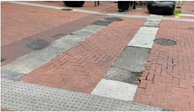
Typical condition of granite pavers. The broken pavers have been replaced with asphalt patches. The asphalt patch is not an effective edge restraint for the brick paving field so the forces acting upon the brick cannot be adequately resisted and the brick within the field of pavers have begun to deflect and move.
