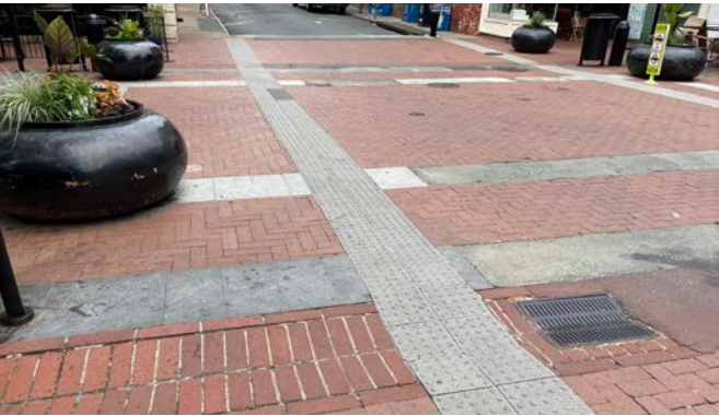
Tactile warning Pavers (12"x12") adjacent to the 2nd Street East crossing. Note the condition of the tactile warning pavers in comparison to the granite bandings which run perpendicular to the flow of traffic. The granite banding is subject to substantially more frequent vehicular loads but also different loads than the tactile warning pavers.
