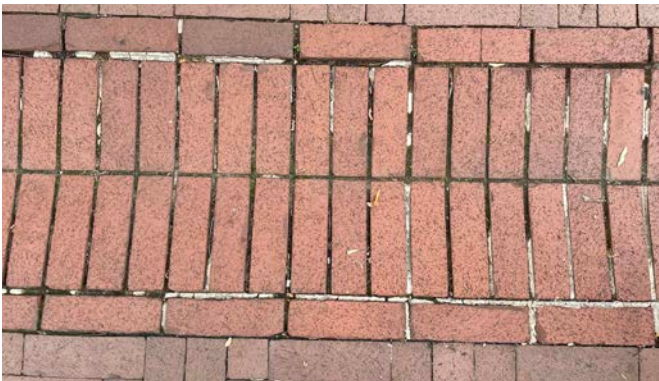
Photo represents the typical condition of the runnels on the downtown mall. Note the lack of mortar remaining between the original brick. (This photo was taken of a drainage runnel along the mall and not within the vehicular crossing because the vehicular crossing runnels have been covered with asphalt).
