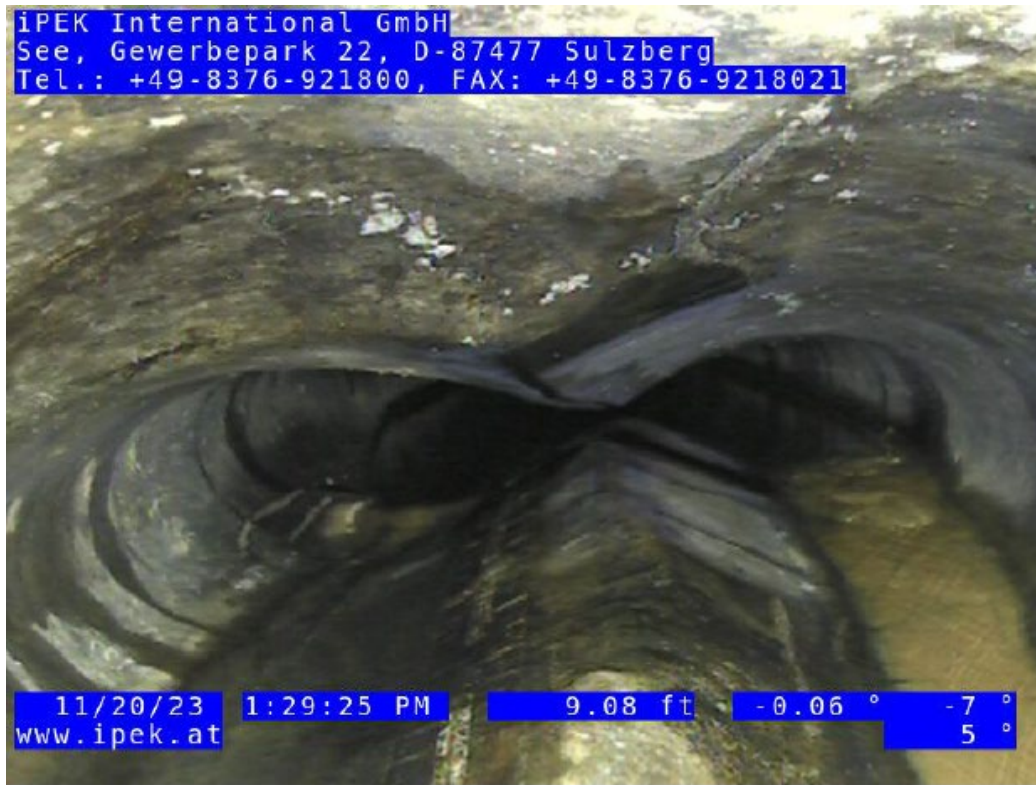
Figure 21 - CCTV image downstream of a crushed pipe along the cemetery road adjacent to Elliott Avenue.
