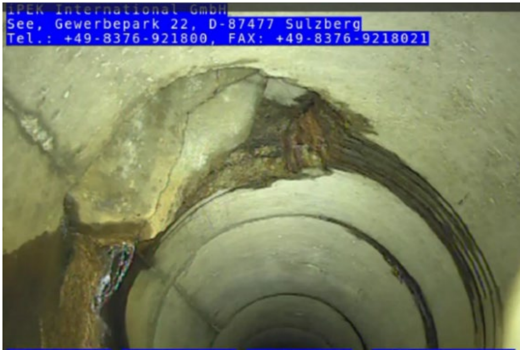
Figure 23 - CCTV Image within the 36-inch RCP pipe along Elliott Avenue. The blind pipe connection leading to the French drains within the Cemetery can be seen within the center of the frame.
