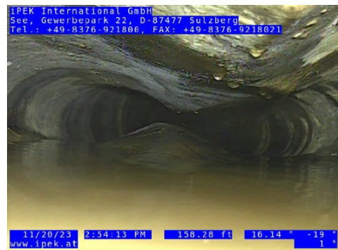
Figure 20 – CCTV image upstream of a crushed pipe along the cemetery road adjacent to Elliott Avenue. Note the volume of water in the pipe.
