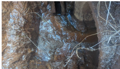
Figure 24 – An earthen manhole type structure connecting the French drains within the cemetery to a pipe which will connect with the 36-inch RCP in Elliott Avenue shown in Figure 21.
