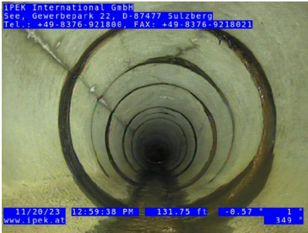
Figure 22 – CCTV Image within the 36-inch RCP pipe along Elliott Avenue. Note the wet seams along every pipe joint.
